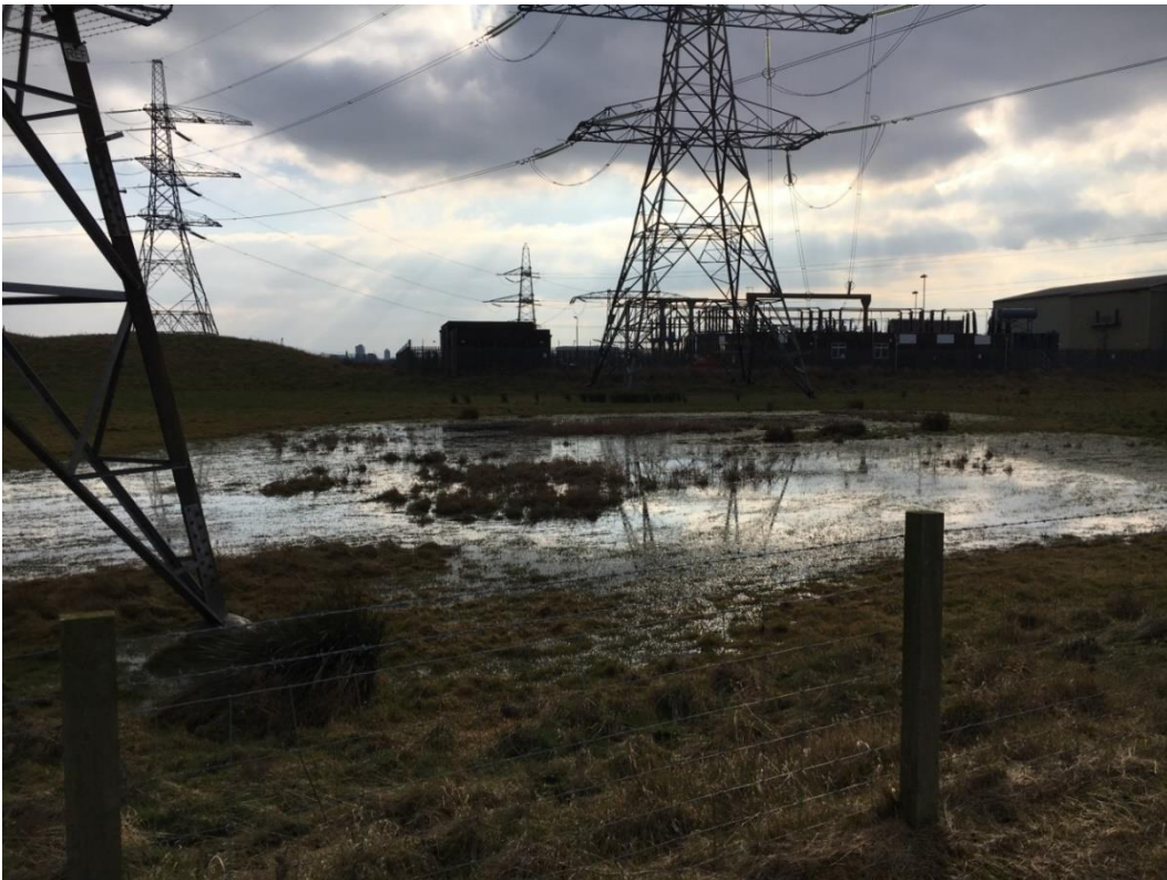
Photograph 18. Inundation area in pasture at Saltholme Substation
